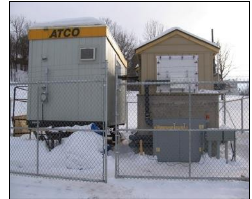
Radon Test Facility
