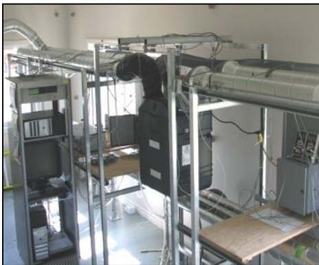
HRV/ERV Test Rig
